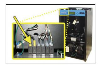
6.5.12.2 Use a Voltmeter to measure the voltage by placing the probes between the Circuit Breaker and terminal insulation so that they touch the metal contacts.
