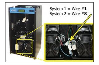
**9.2.3** Use an Amp Meter to measure the running amps.
