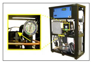
**8.15.4** With a 3/8" wrench, turn the adjustment screw on the Valve in 1/4 turn increments until 35° - 45°F is indicated on the **RRU TMP** of the display screen.
