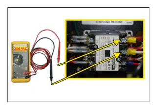
Voltage From To Black 208 - 230 VAC P20KW L1 L2 White 208 - 230 VAC L1 Black L2 White 208 - 230 VAC P30KW L1 Black L3 Red L2 White L3 208 - 230 VAC Red
