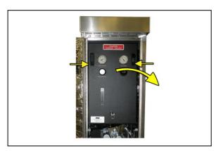
**8.4.3** Remove wing nut and washer. Open Top Cover.
