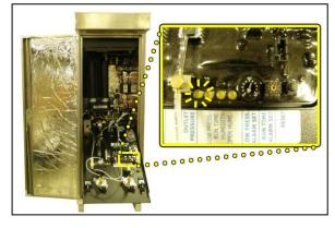
**9.15.7** Press the **RESET Button** to clear the Humidity alarm.
