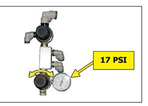
6.5.27.2 Turn knob untilOutlet Pressure(OUTLET) reading is at the desired setting.
