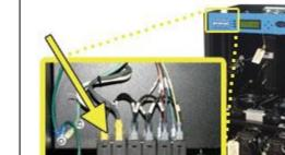
6.5.12.2 Use a Voltmeter to measure the voltage by placing the probes between the Circuit Breaker and terminal insulation so that they touch the metal contacts.
