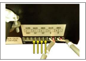
11. Route Alarm cables **A** and **B** into dryer and install to the alarm points. A is "MINOR IN" alarm; **B** is "MAJOR IN" alarm.
