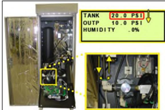
**9.11.6** Verify the compressor turns on when the tank pressure (**TANK**) falls to **20.0 PSI**.
